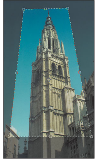
Figure 2.12 Drag the side, top, and bottom handles to enlarge the area to be fixed.
